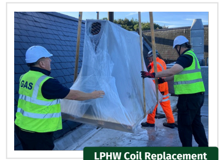
LPHW Coil Replacement
